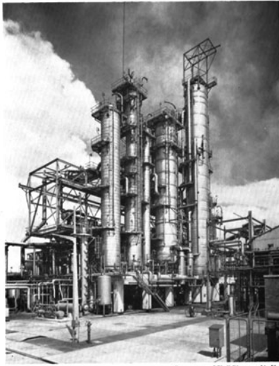
By courtesy of Shell Photographic Unit This refinery and chemical plant at Shell Haven makes lubricating oils, bitumen, paraffin wax, gasoline, diesel oil, gas oil, fuel oil, bottled gas, refinery gas, ammonia, fertilisers, insecticides, detergents, alkylates, sulphur and many other products.
